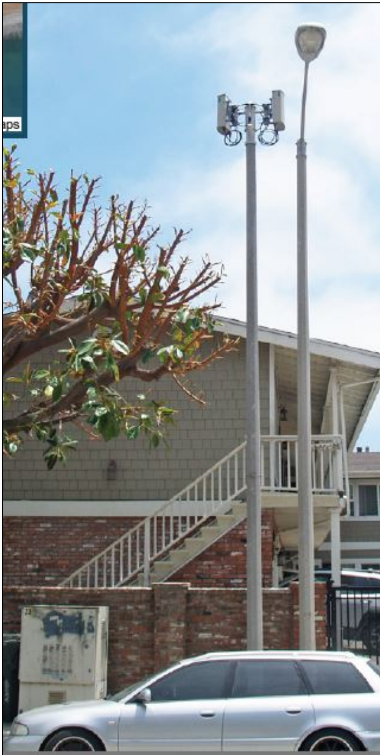
Figure 2: Existing antennas on Pole and ground-mounted meter cabinet (Source: Applicant submitted Photo Simulations).
