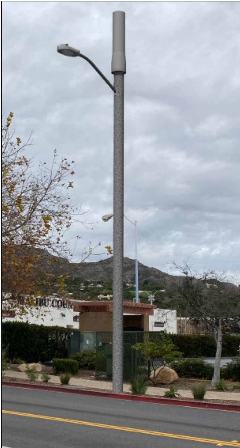
Figure 3: Photo simulated view of node on Pole. (Source: Applicant submitted Photo Simulation).
