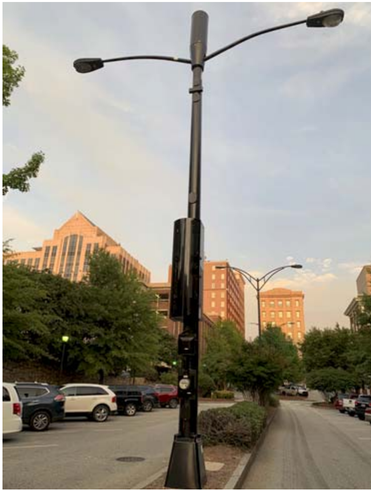
Example of a Small Cell Installation
