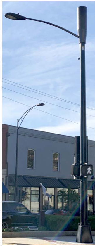
Example of a small cell installation.
